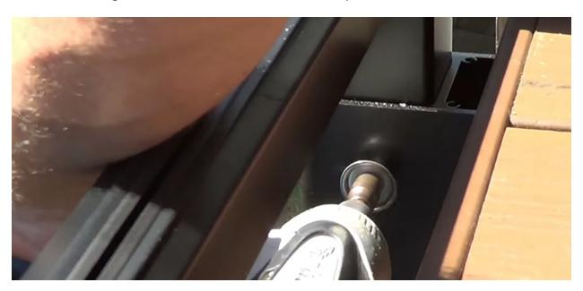
**Step 15:** Secure the bottom rails by installing the self drilling screws on the outside surface of each end of the rails.
