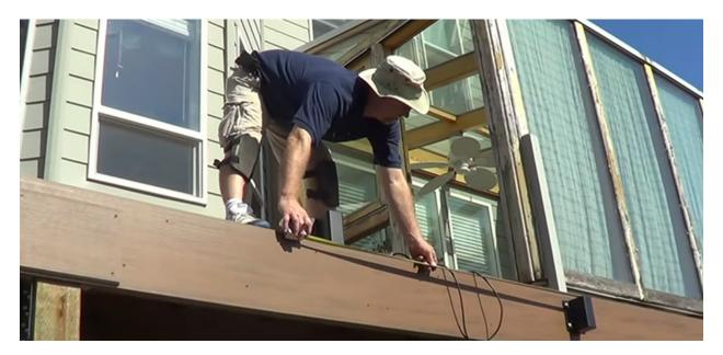
**Step 2:** Install the fascia brackets by first drilling a 1/4'' inch diameter pilot hole, and then install the 43/8'' lag screws per bracket. Be sure to include the stainless steel cupped washers on each lag screw.
