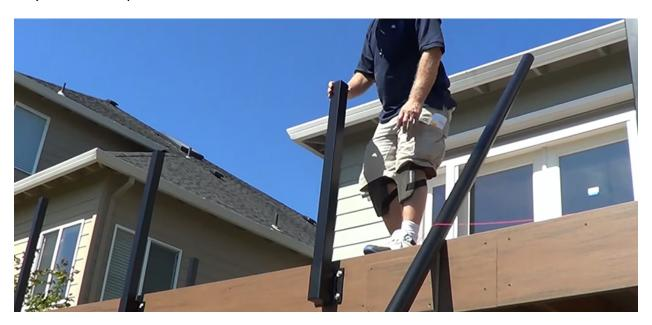
**Step 6:** Install the top rail brackets. For the corner posts, remove the perforated tabs.
