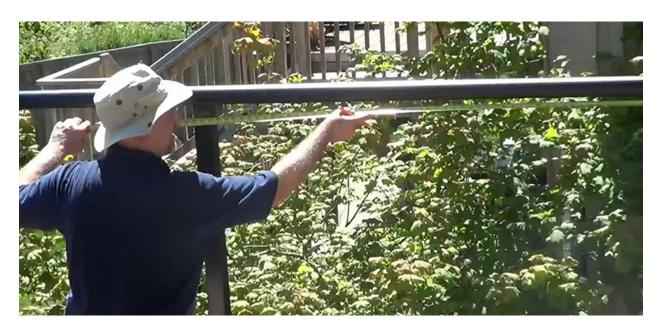
**Step 13:** Snap the top rail glass infill into the underside of the top rail.
