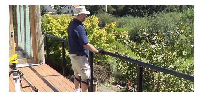
**Step 9:** Install the self drilling screws through the underside of the top rail brackets to secure the top rail.
