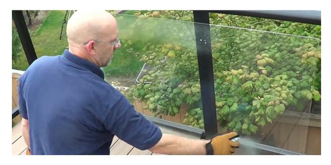
**Step 17:** Insert the top of the glass panel into the top rail. Be sure to push the glass all the way up into the channel. Then insert the bottom of the glass into the bottom rail and centre the panel between the posts.
