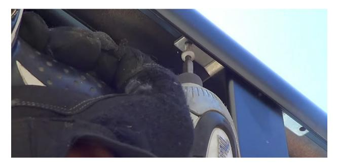
**Note:** If you have a run of top rail longer than 20 feet, you'll need to splice two top rail sections together. To ensure a tight splice, use a ratchet strap to pull the top rails together, and secure with the splice plates and self drilling screws.
