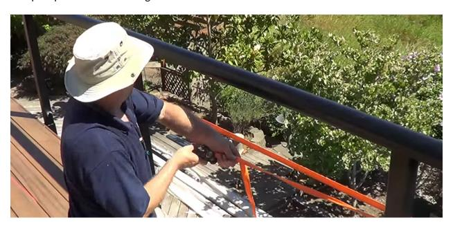
**Step 10:** Using your tape measure, mark the posts where the bottom rail connecting blocks will be installed.
